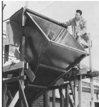
Ewen's horn antenna mounted on the Lyman Physics Lab at Harvard. The dielectric window was installed to keep rain from flooding the lab, and deflect snowballs thrown by Harvard students.
